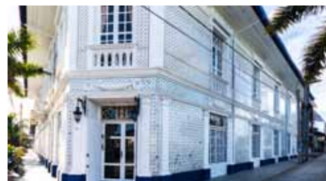
Casa Morey MID-RANGE
